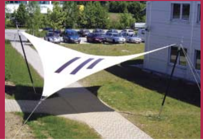
Four point sail with PV Flexibles as entrance canopy
